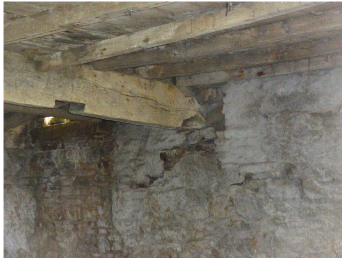
Figure 12 - deflected/failed beam
