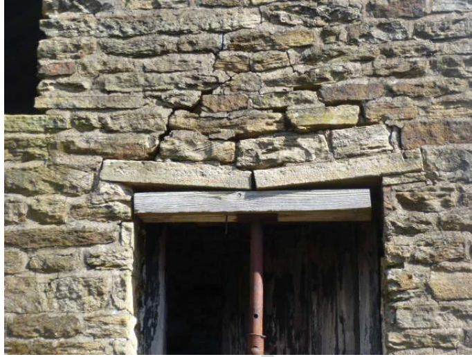
Figure 2 - failed lintel
