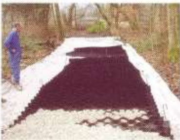
CellWeb during installation.
