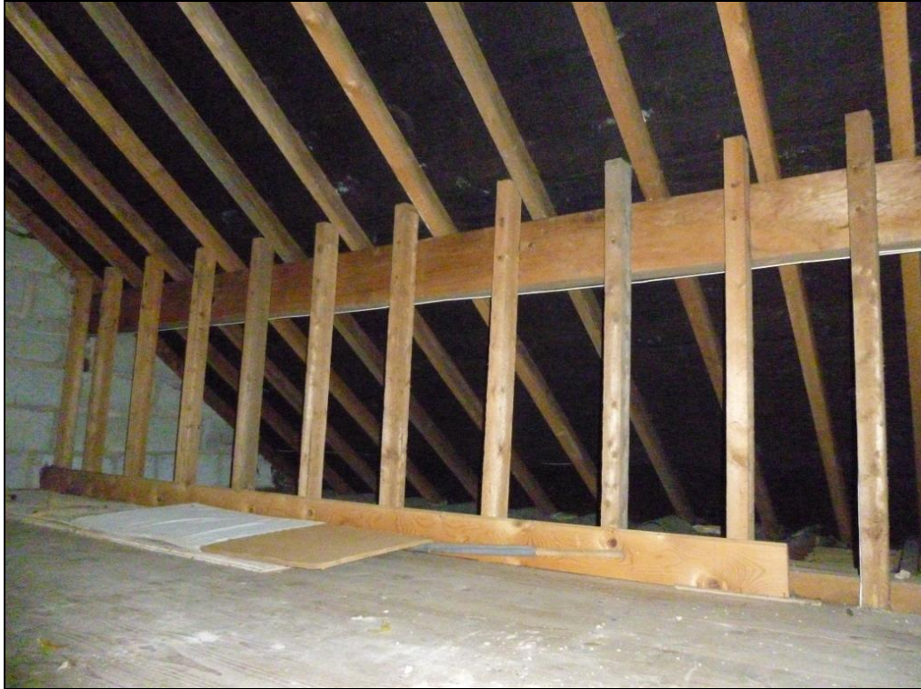
Photograph 7 showing internal view of loft space
