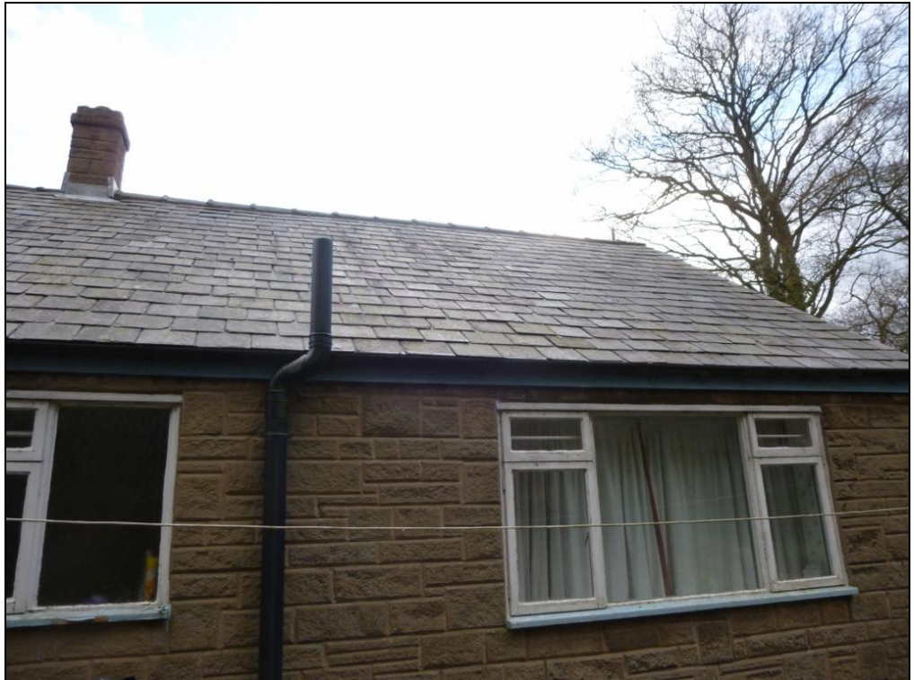
Photograph 3 showing the rear of the property, including the roof
