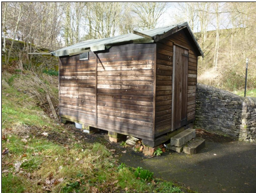
Photograph 6 showing wooden shed at the rear of the property.
