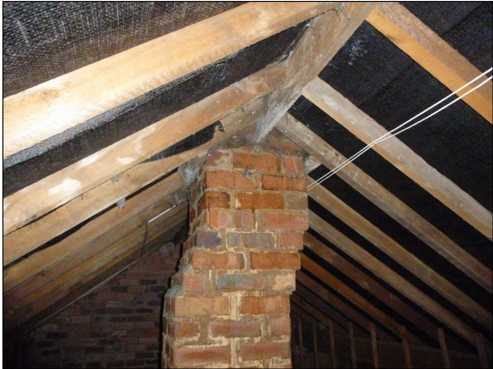
Photograph 9 showing the chimney stack and brickwork gable end
