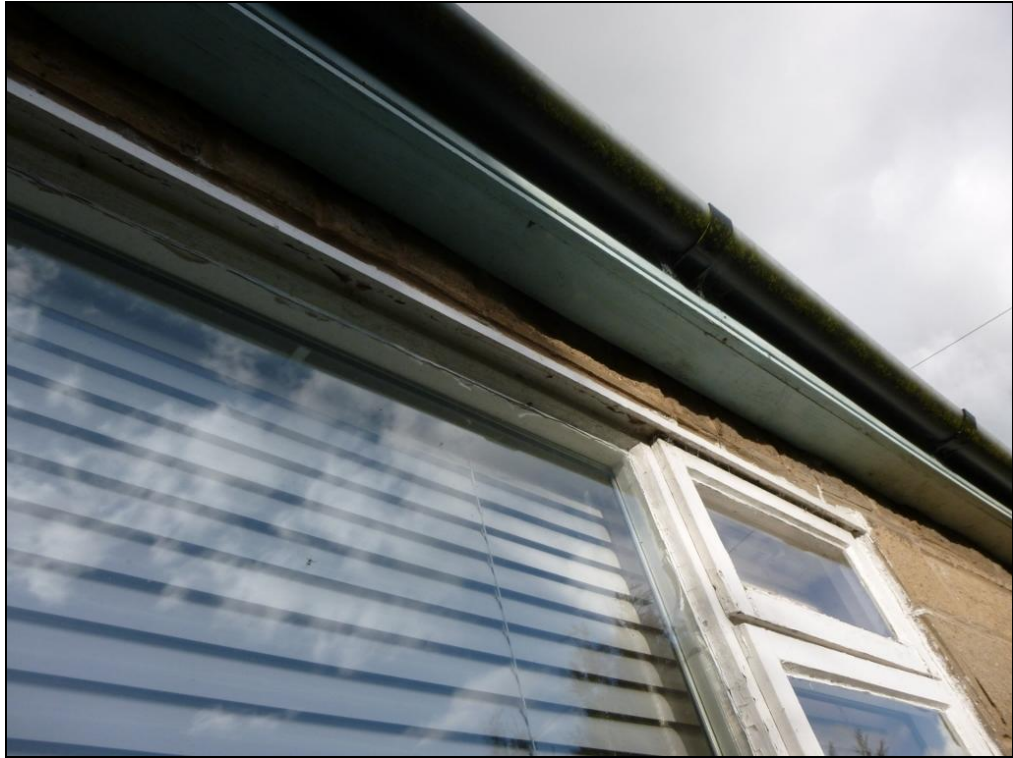
Photograph 4 showing the wooden soffit boxes and barge boards in good condition
