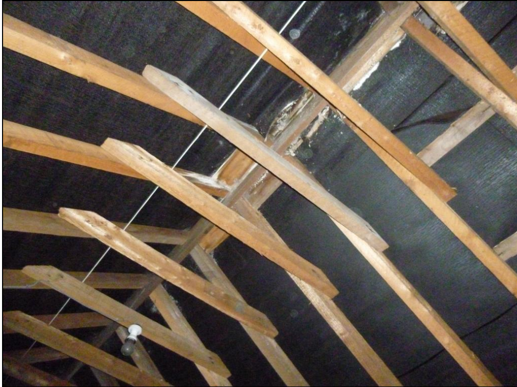
Photograph 8 showing the good condition of the roof felt and joists
