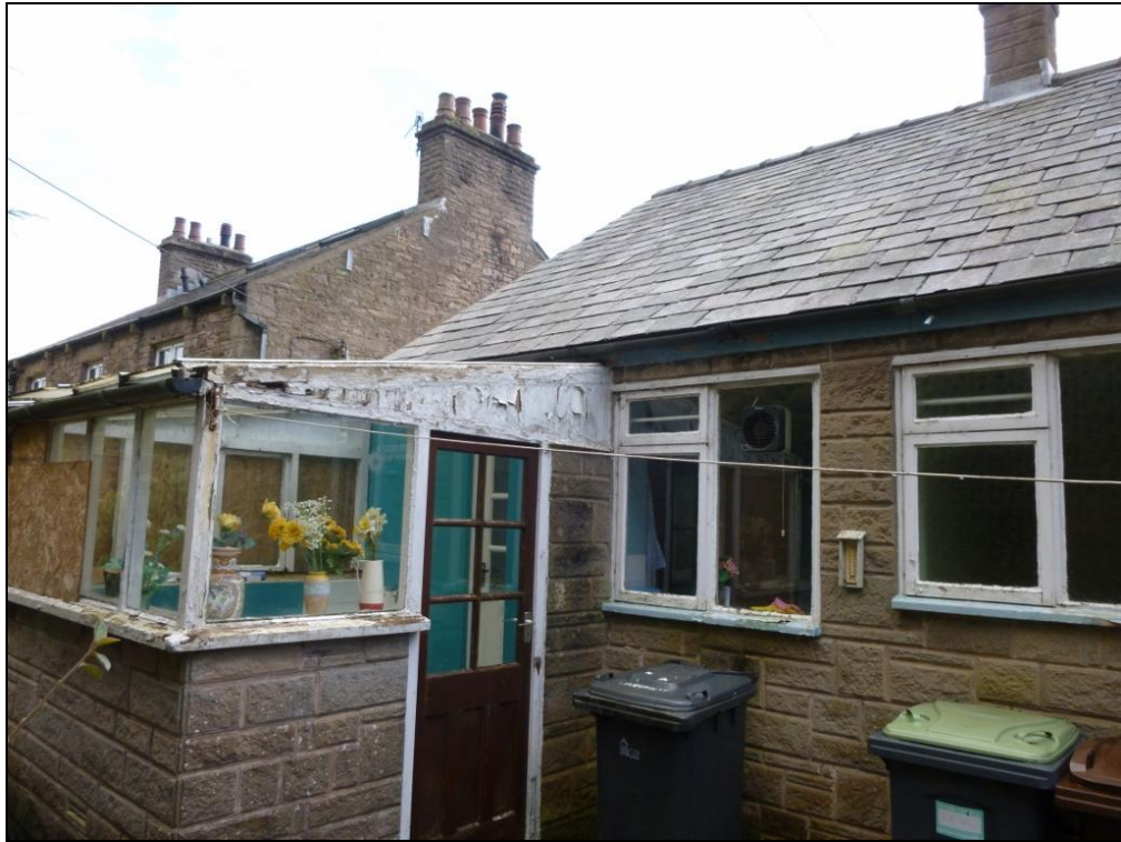
Photograph 5 showing wooden frame lean-to at the rear of the property
