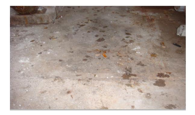
Condition of asbestos insulation debris to Area 3 - Tank Room.
