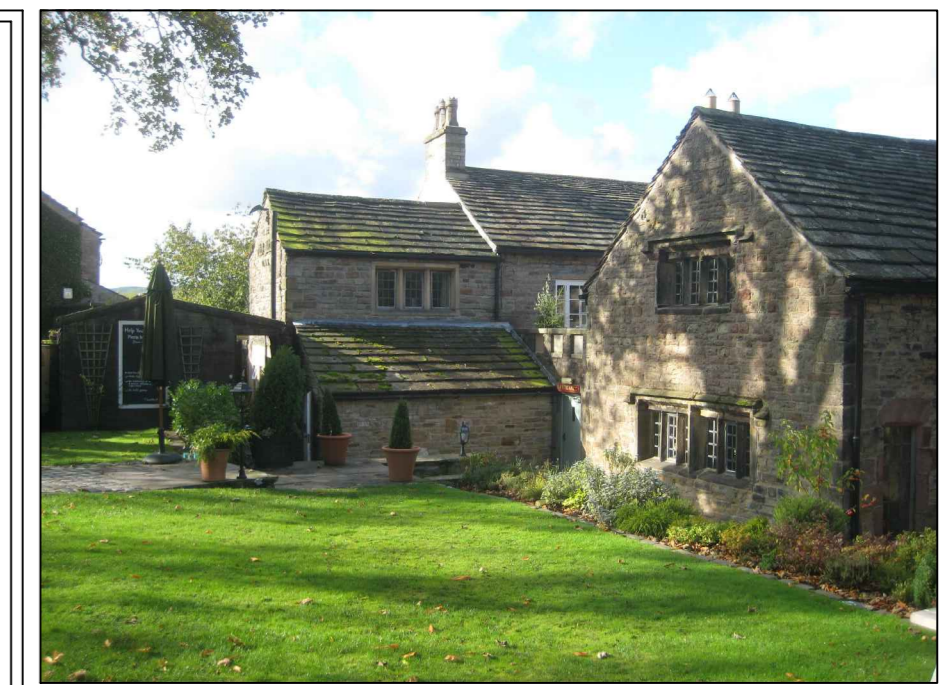
South and East Elevations
