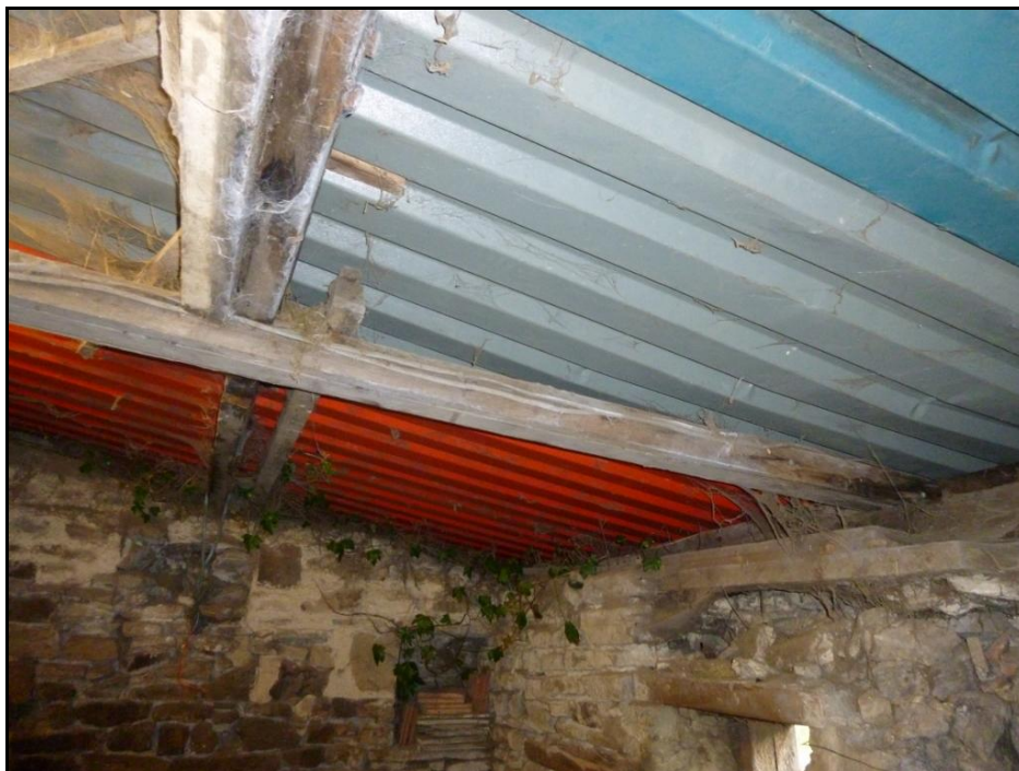
Photograph 6 showing the internal corrugated metal roof
