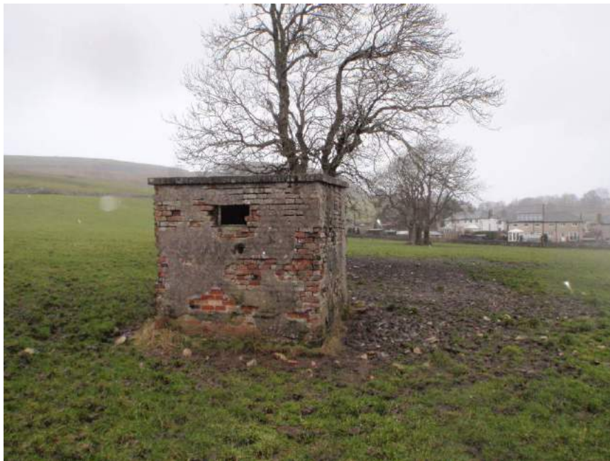
Plate 10 Southern part of site, small brick shed near centre of area, looking northwest
