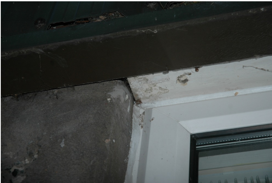
Figure 5. Details of crevice above window frame – left side
