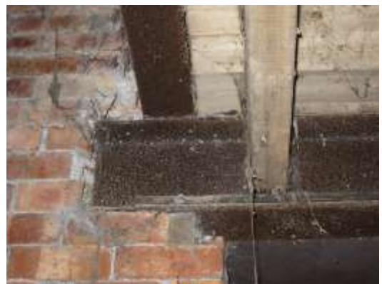
fig 12) undersized steel- sag
