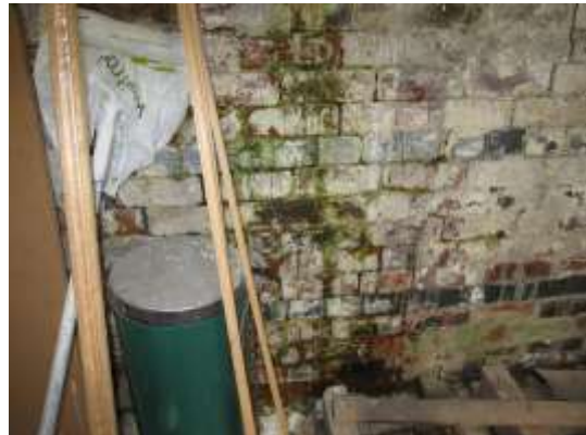
fig 18) damp penetration
