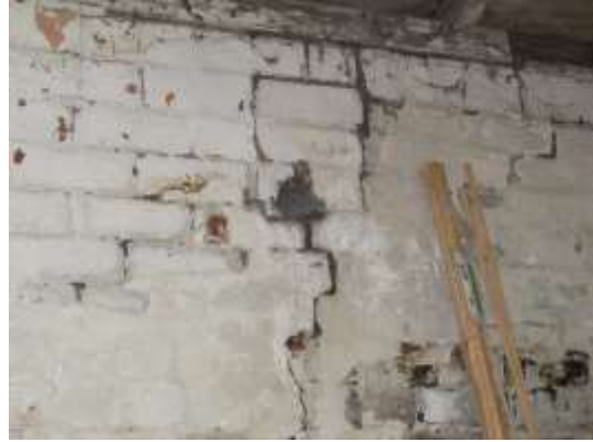
Fig 16) settlement cracks
