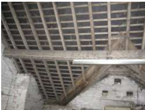
Fig 19) undersized purlin
