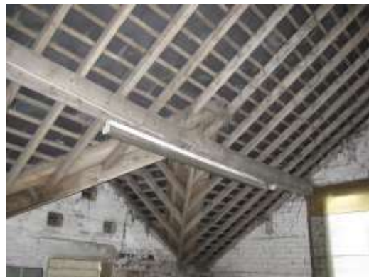
fig 20) undersized purlin
