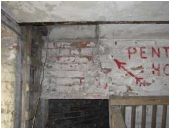
Fig 29) settlement around door
