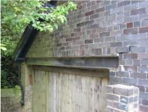
Fig 3) lintel needs replacing
