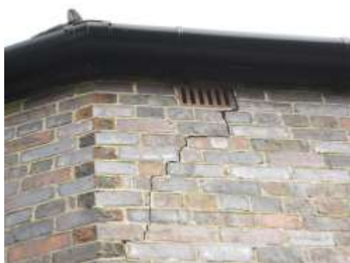
Fig 23) undersized beam
