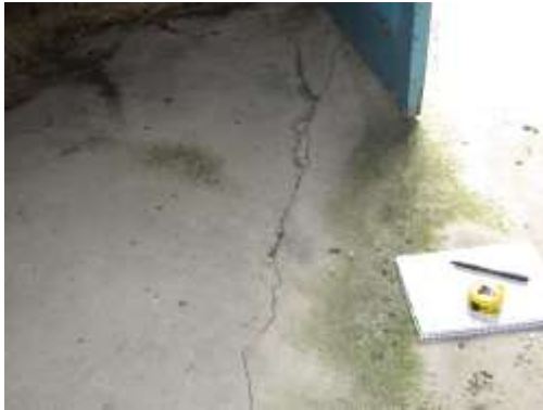
Fig 27) first floor crack in slab
