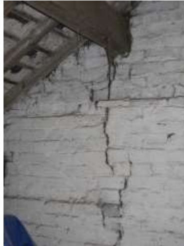
Fig 22) settlement crack
