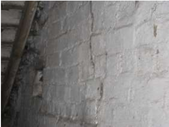
Fig 21) settlement crack
