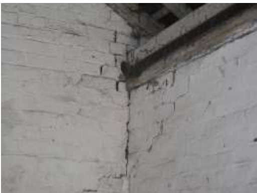
Fig 7) separation at corner
