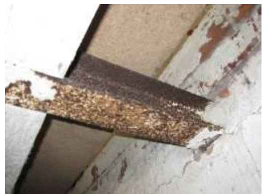
fig 8) filler joist floors
