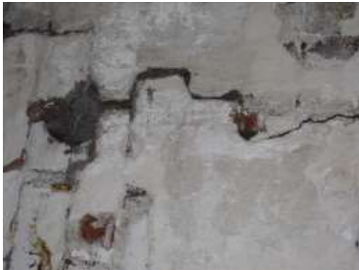
Fig 17) settlement cracks
