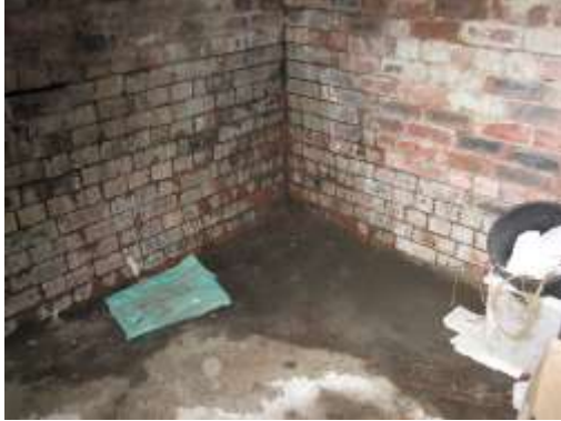
Fig 9) damp penetration
