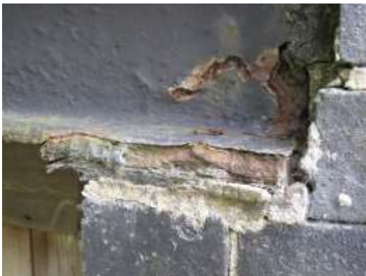
Fig 1) corrosion of lintel bearing
