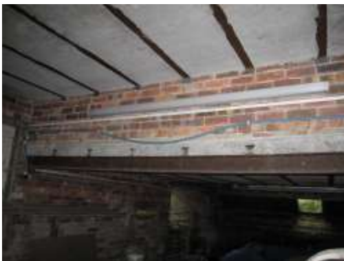
Fig 23) undersized beam
