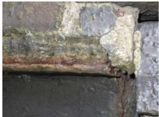
fig 2) lintel bearing area
