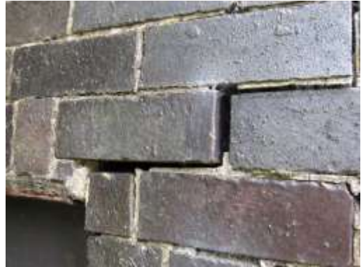
fig 4) damage due to lintel
