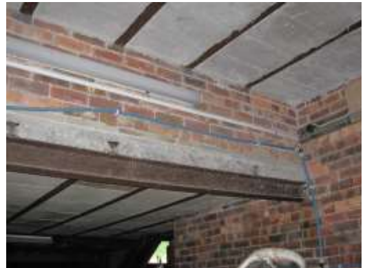
fig 12) undersized steel- sag
