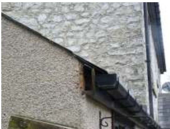
Plate 2; showing crevice leading into the lower ground roof void indicated by the red arrow.
