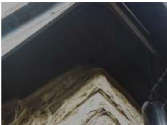
Plate 3: showing soffit box with crevice suitable for bat access into main roof void within the house.
