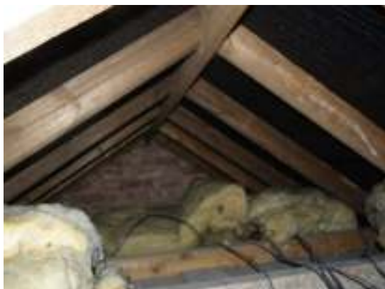
Plate 4: Showing internal view of the lower ground roof void, showing tightly fitted roofing felt which could not be fully inspected.
