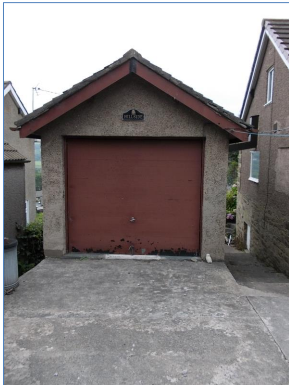
Figure 6: South elevation of garage (building B2).
