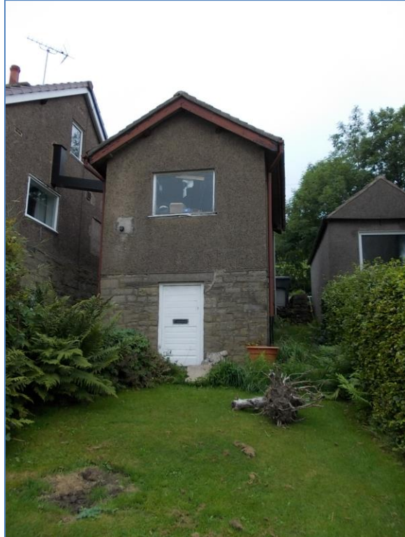
Figure 5: North elevation of garage (building B2).
