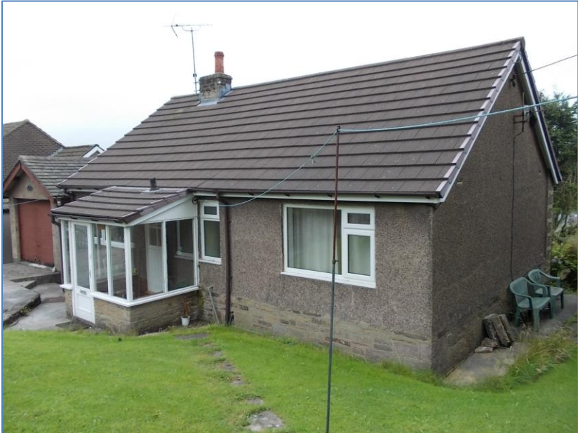
Figure 2: South elevation (building B1).
