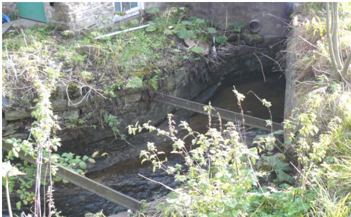
Photo. 7: Water entering the culvert that passes under the Site's access road
