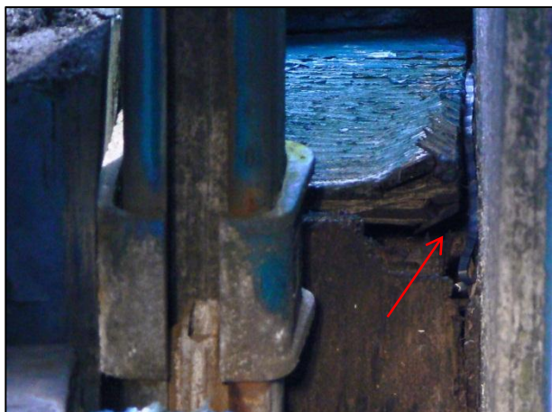
Photograph 7: Rot hole in frame of sliding door
