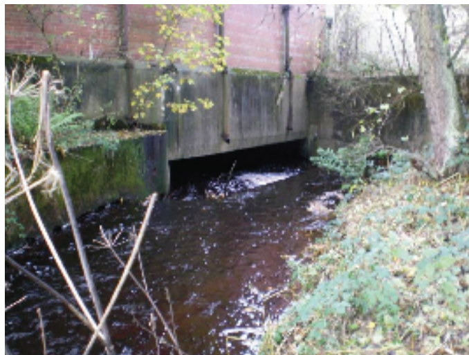
Upstream culvert entrance under Building 1
