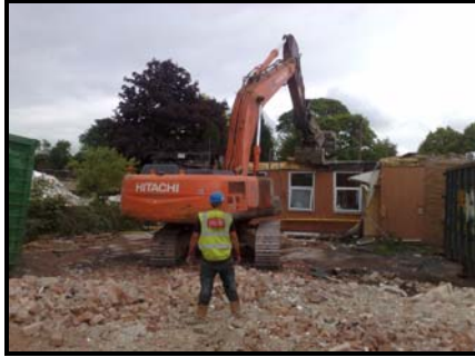
Photo shows demolition type excavator fitted with grapple type attachment.
