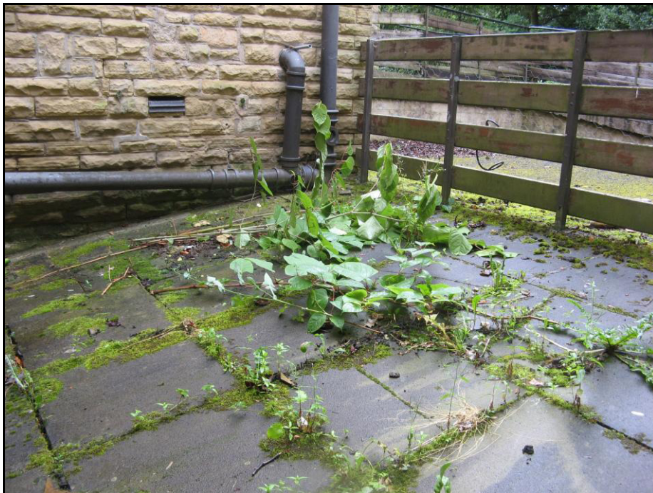
Photograph 5 showing Japanese Knotweed growing out the flags along the western edge of the building (near to cellar entrance)
