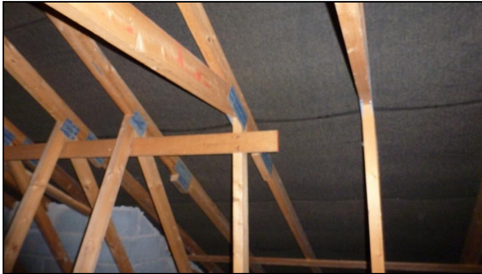
Photograph 7 showing good condition of felt roof lining and timber joists
