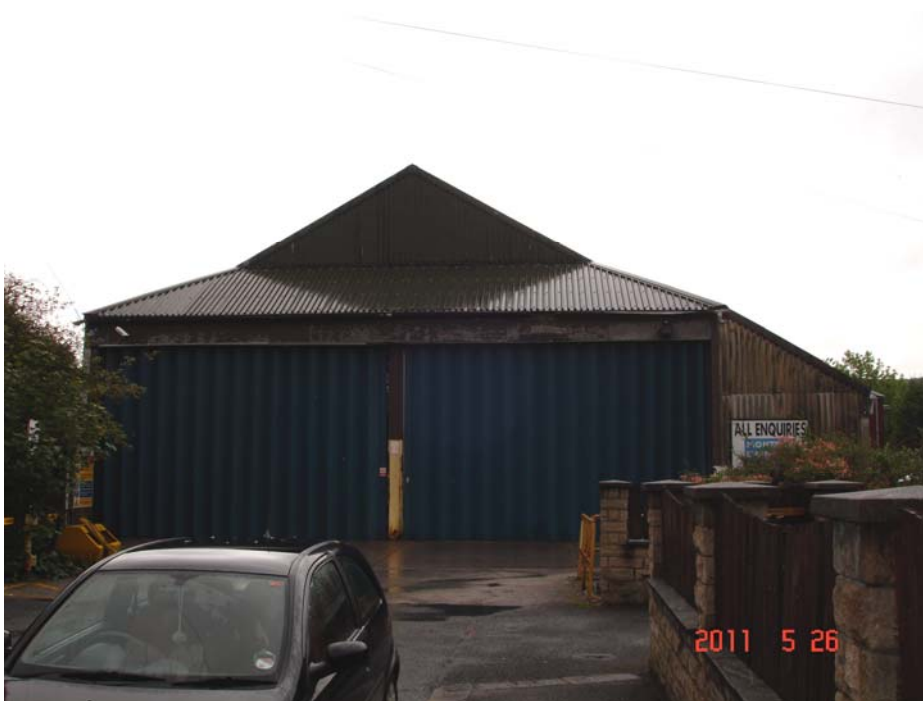
Front elevation of bus depot.
