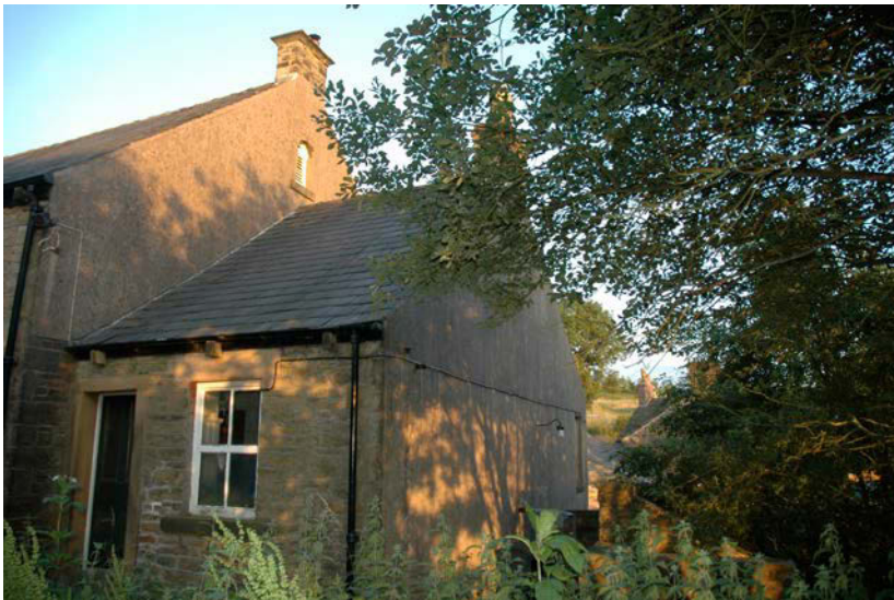
Figure 4. West end of Brookbottom Methodist Church.
