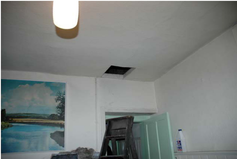
Figure 13. Entry hatch to vestry attic space, Brookbottom Methodist Church.
