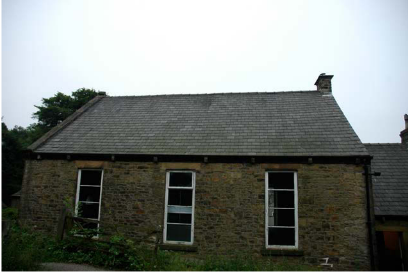
Figure 5. North side of Brookbottom Methodist Church.
