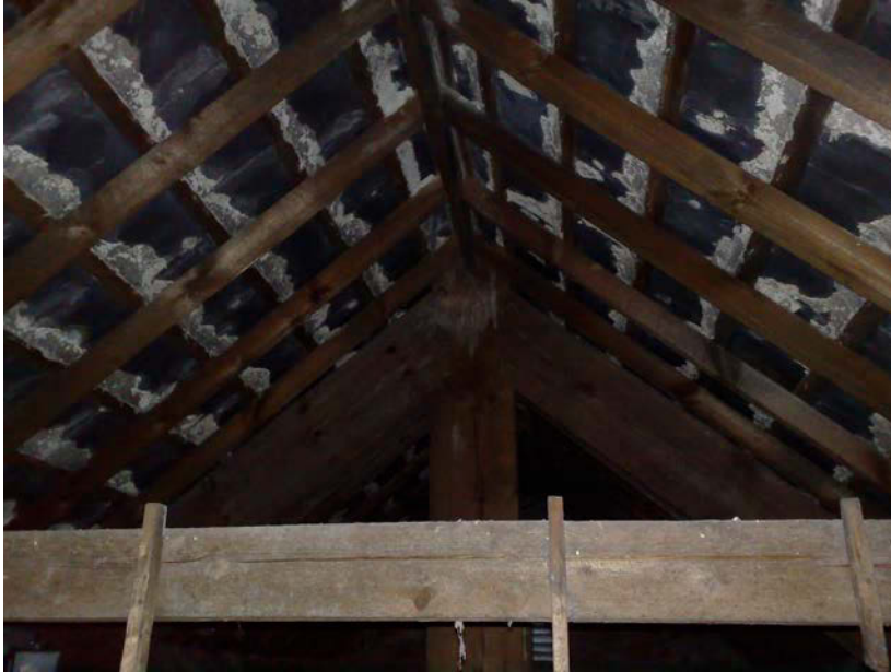
Figure 9. Church attic space
