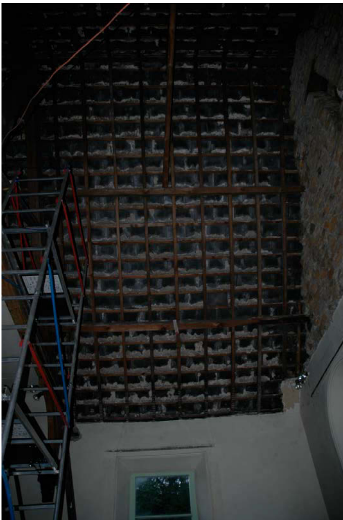
Figure 12. Internal view of roof at Brookbottom Methodist Church.
