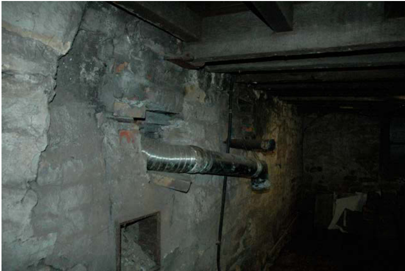
Figure 7. Cellar space at Brookbottom Methodist Church.
