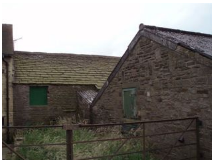
Photo 5. The barn and shippon as viewed from the northeast
