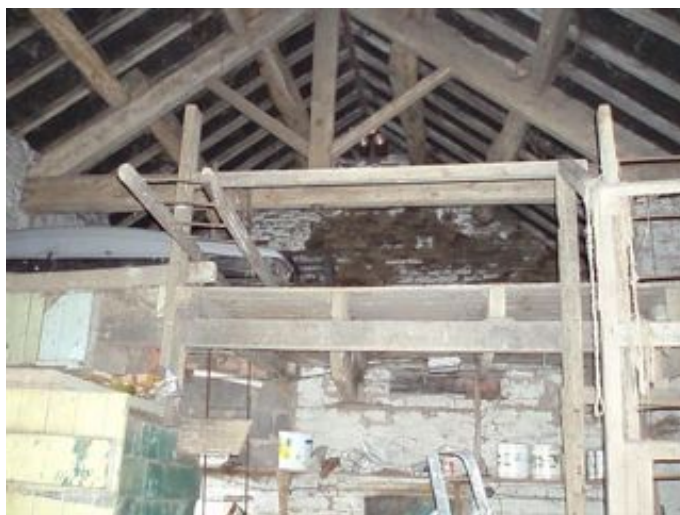
Photo 10. The interior of the barn showing the split loft
