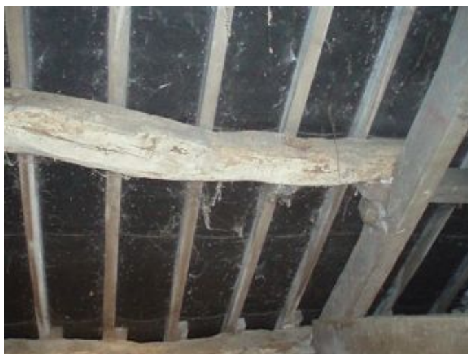
Photo 11. Detail of the roof beams and rafters within the barn
