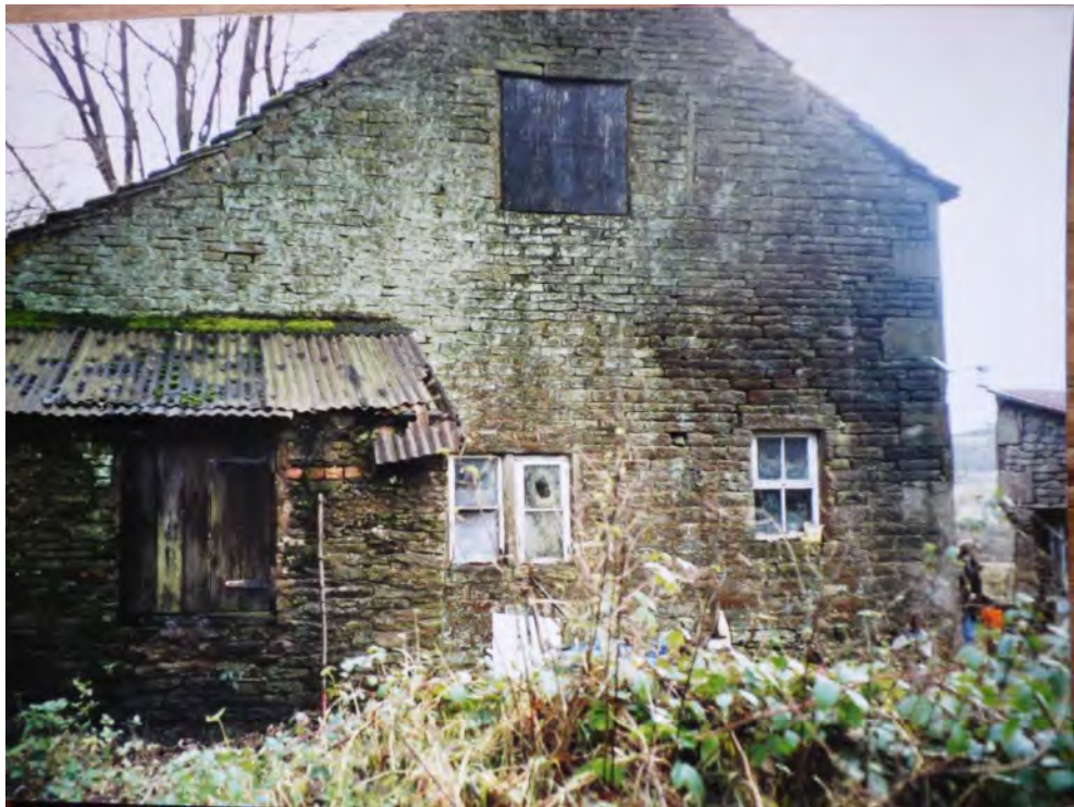
Fig.4 west gable-end with lean-to outhouse, prior to refurbishment
