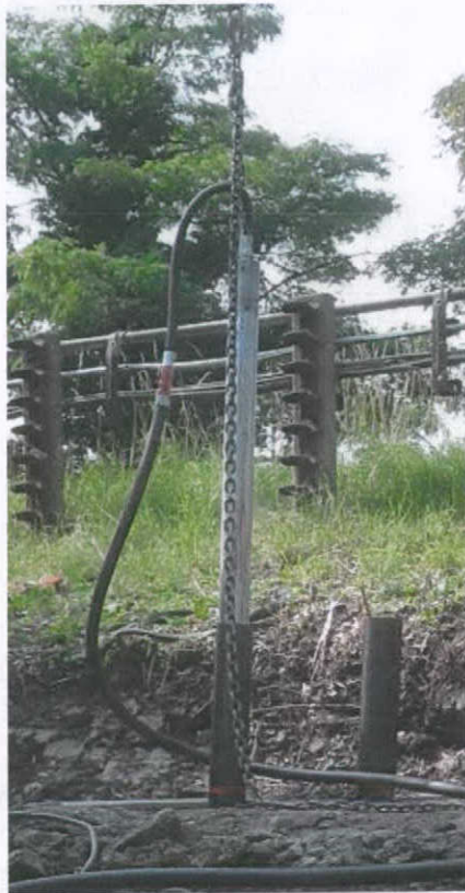
GRUNDOMAT being removed from the pile
