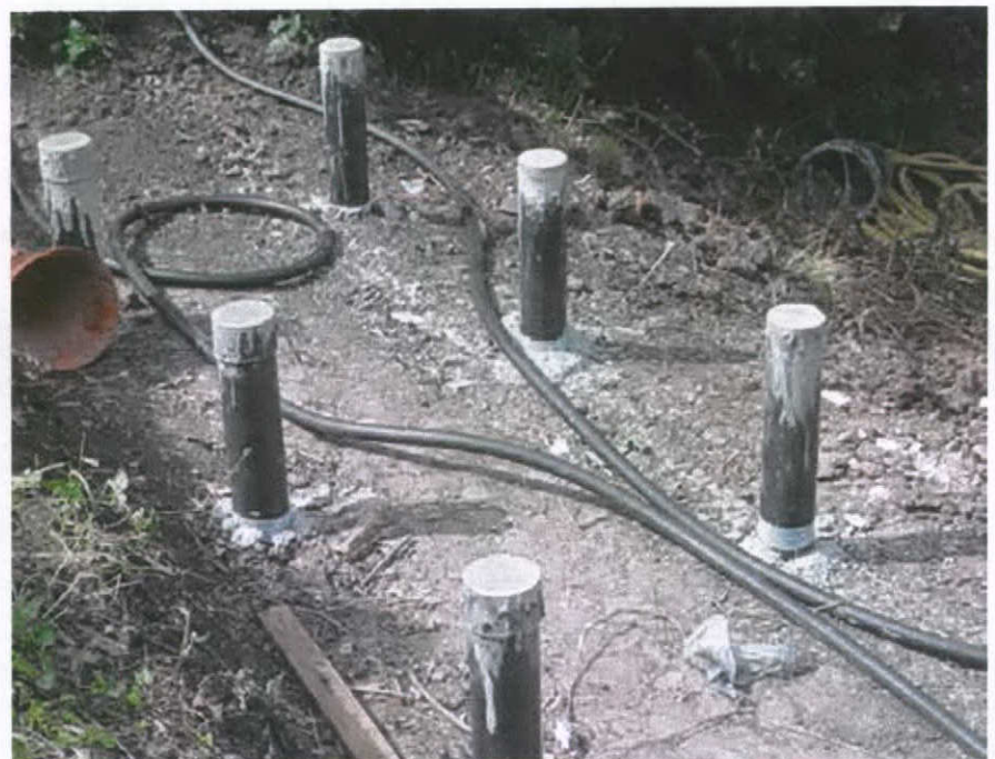
Reinforced concrete piles now firmly in place
