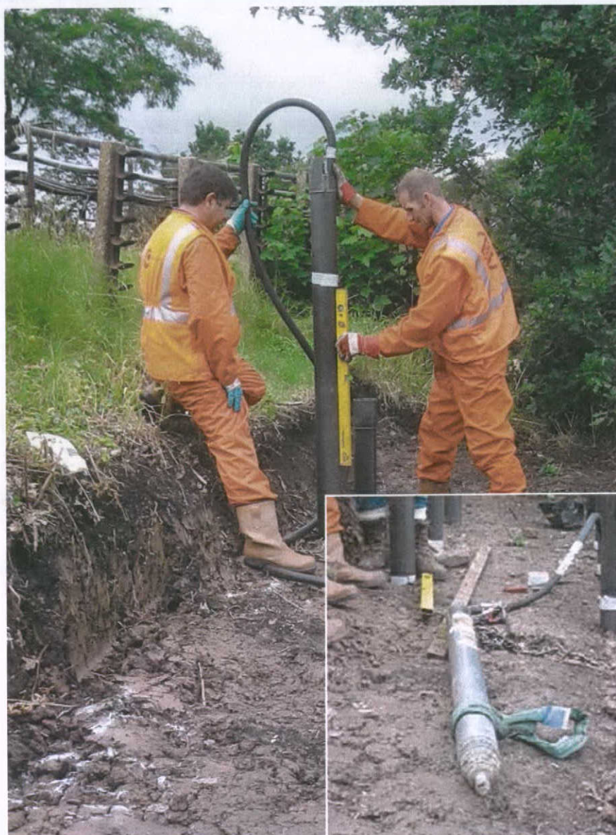
The Operators ensuring the pile is driven plumb by using a spirit level
