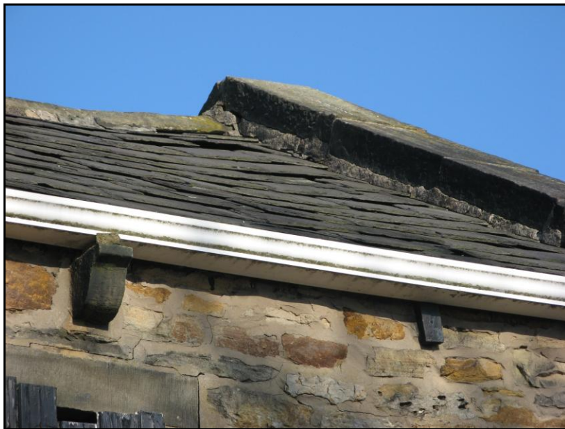
Photograph 6 showing a gap between the slate tiles
