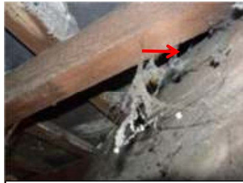
Roof Space 3: potential roosting example
