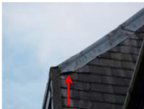
Plate 4: showing potential bat and bird access and roosting potential
