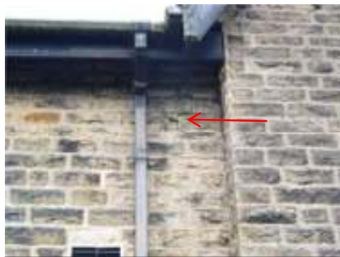
Plate 2: showing potential bat and bird access and roosting potential
