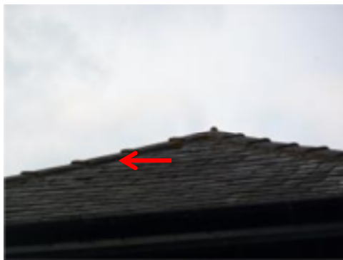
Plate 1: showing potential bat and bird access and roosting potential
