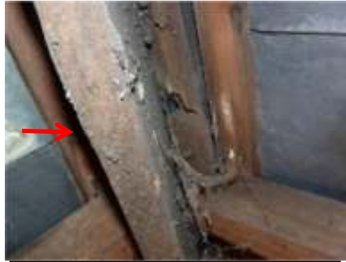
Roof Space 1: example of roosting opportunity.
