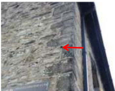
Plate 3: showing potential bat and bird access and roosting potential
