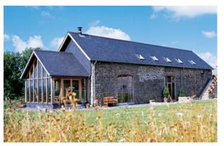
The gable extension demonstrates that the use of vertical glazing panels with a slate roof can ensure a sensitive but clearly contemporary addition to a traditional building.
