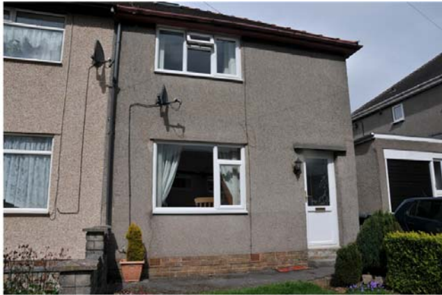
ES01. FRONT OF EXISTING DWELLING
