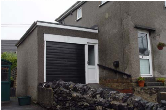
ES07. SE SITE BOUNDARY - ALONG WALL & GARAGE TO NO. 13
