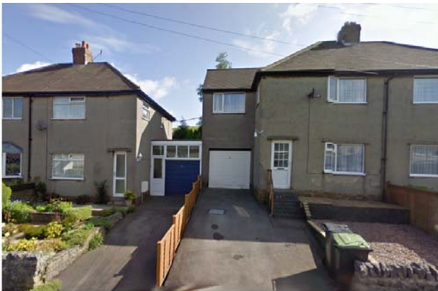
EA05. VIEW OF NO. 29 - FEATURING SIMILAR 2ST EXTENSION
