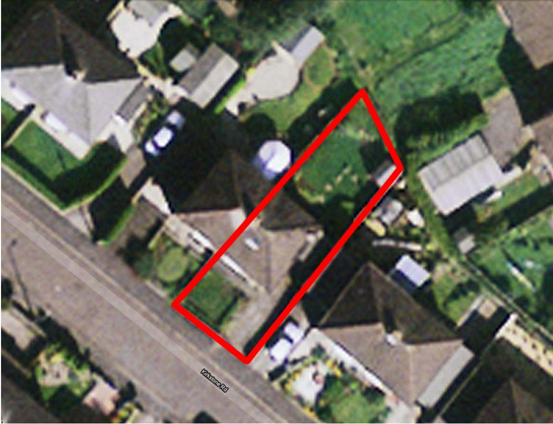
Aerial view of the site showing the site boundary
