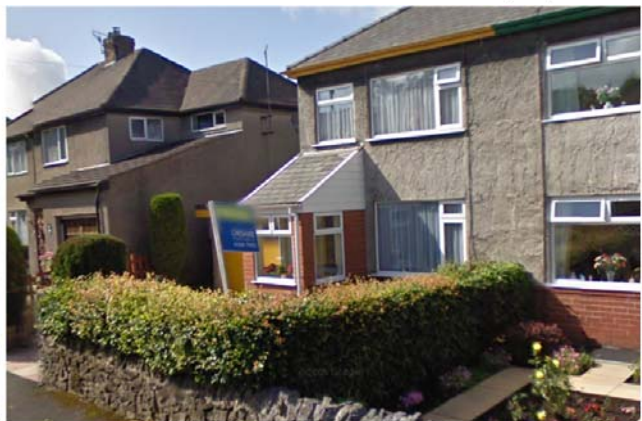
EA04. VIEW OF NO. 20 - FEATURING BRICK & TIMBER EXTENSION
