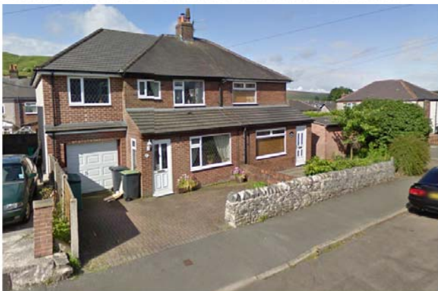
ES07. VIEW OF NO'S 4&2 FEATURING BRICK EXTENSIONS
