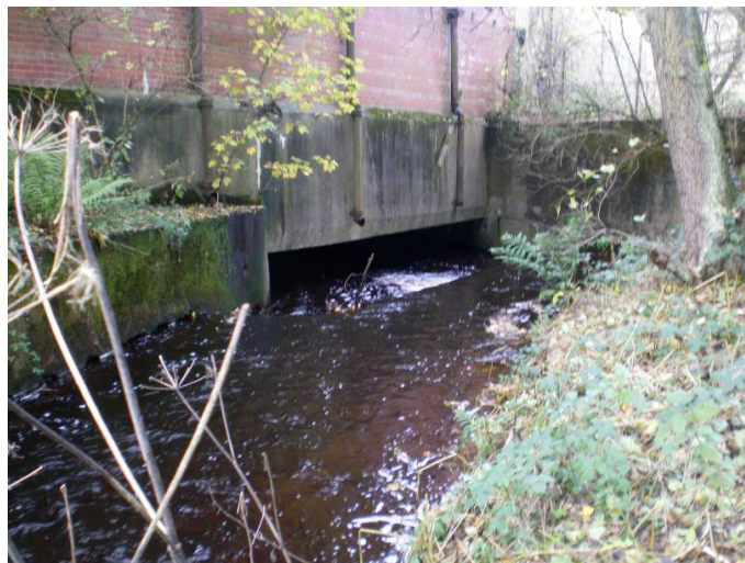
Upstream culvert entrance under Building 1
