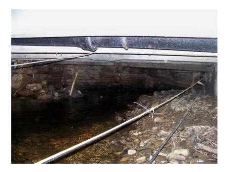
2.2.3. Within the culvert there was an accumulation of debris that suggests that the water depth in the culvert will rise at times of high flow making the walls unsuitable for roosting or hibernating bats.
