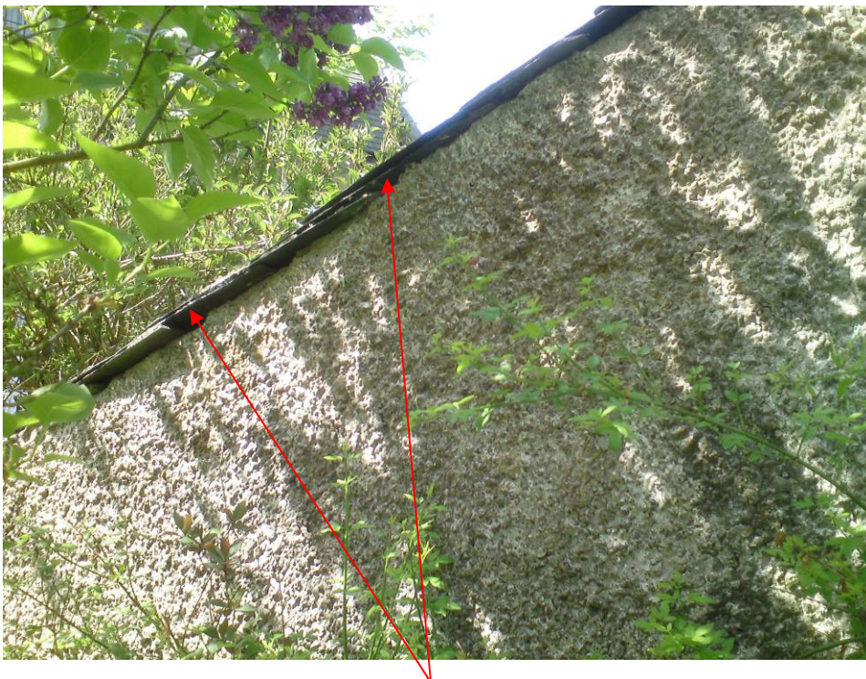
Minor gaps at east verge where gaps should be immediately sealed
