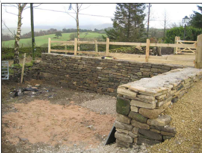
New retaining wall adjacent to proposed shed
