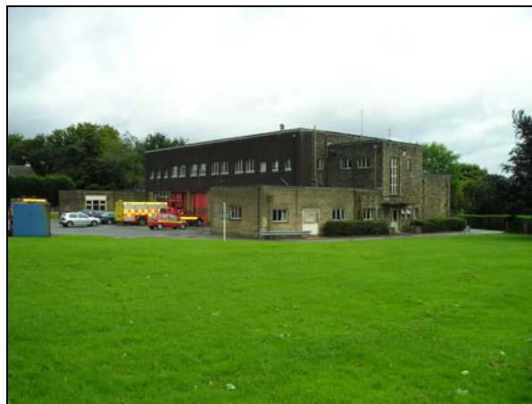
Plate 4 – Facing the rear of the main station building (southern aspect)
