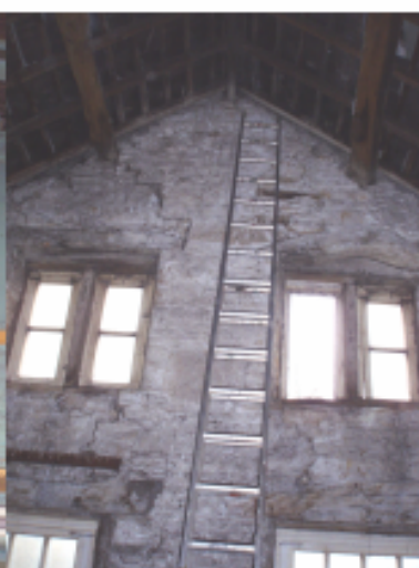
P5 Top floor, building 3
