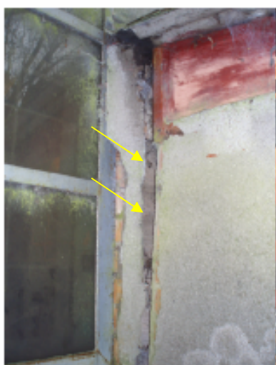
P3 Gap buildings 2 and 4
