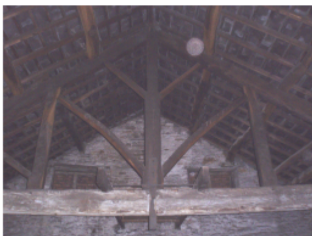
P6 Top floor, building 3
