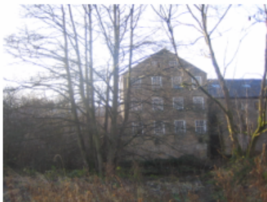
P1 Building 3, N gable
